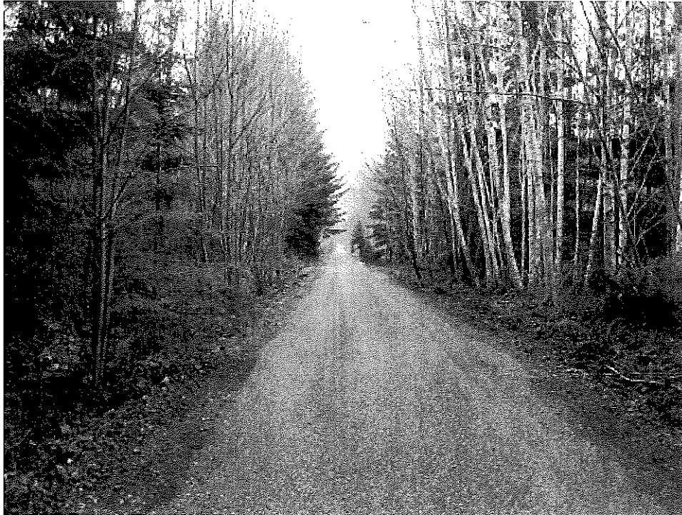
Recently placed ¾" Road Base – Ready for final surface material
