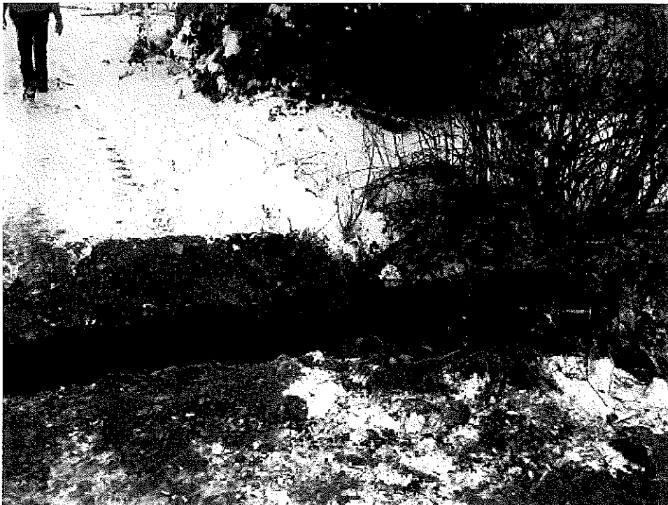
One of four culverts at the marsh flooded by beavers. These near-surface culverts extend into the marsh and the exposed inlet been perforated to allow passage of water even if it is blocked. Their proximity to the trail edge allows for easy maintenance, while their proximity to the trail surface allows the water level to stay at a sustainable level for the beavers.
