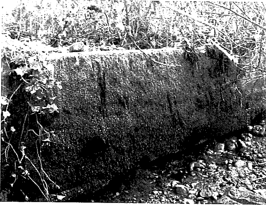
Photograph 5: Concrete weir (1.0 m height) approximately 15 m upstream of stream mouth at Mill Bay
