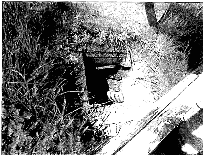
Overflow pipe from the larger pond at the point where it crosses underneath the driveway.
