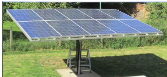
Ground mount installation of solar panels.
