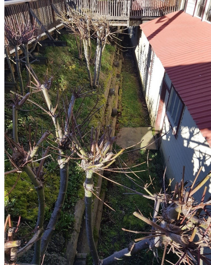
Photo 7: View of timber crib wall supporting Cowichan Bay Road.
