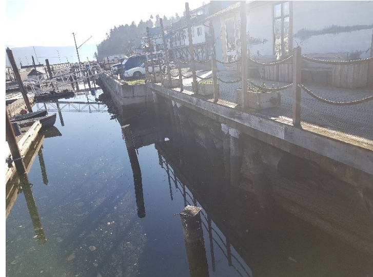
Photo 2: View of existing timber crib and concrete block retaining walls.
