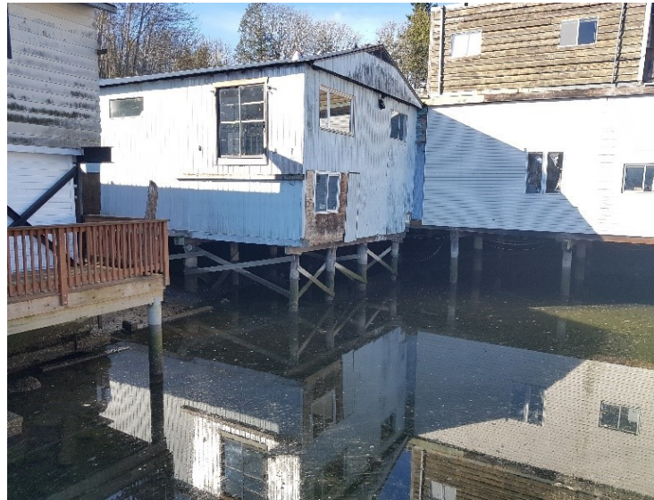
Photo 3: View of existing structures founded on piles.
