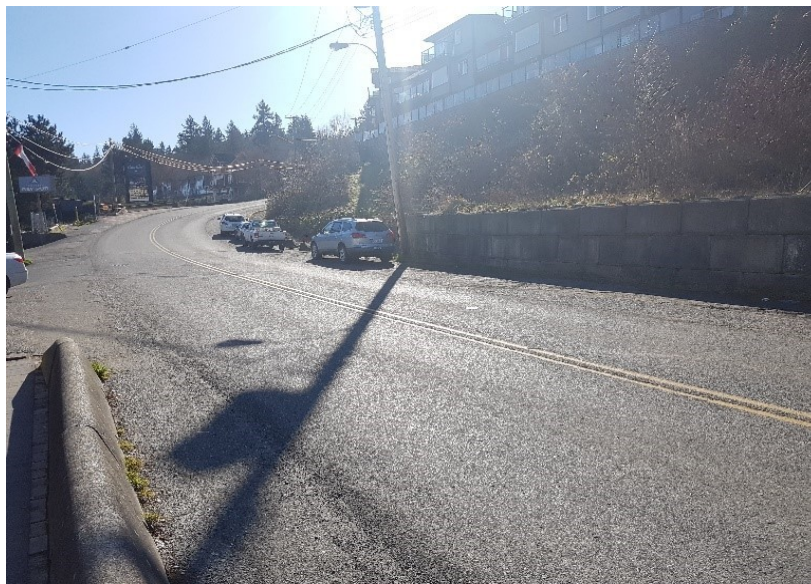
Photo 4: View of Cowichan Bay Road looking east with upslope “lock-block” wall
