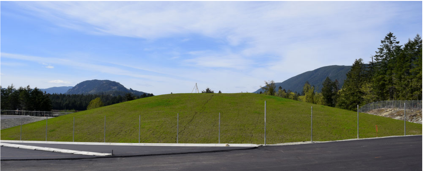
The CVRD Meade Creek Recycling Centre - Encapsulated Garbage Incinerator Ash
