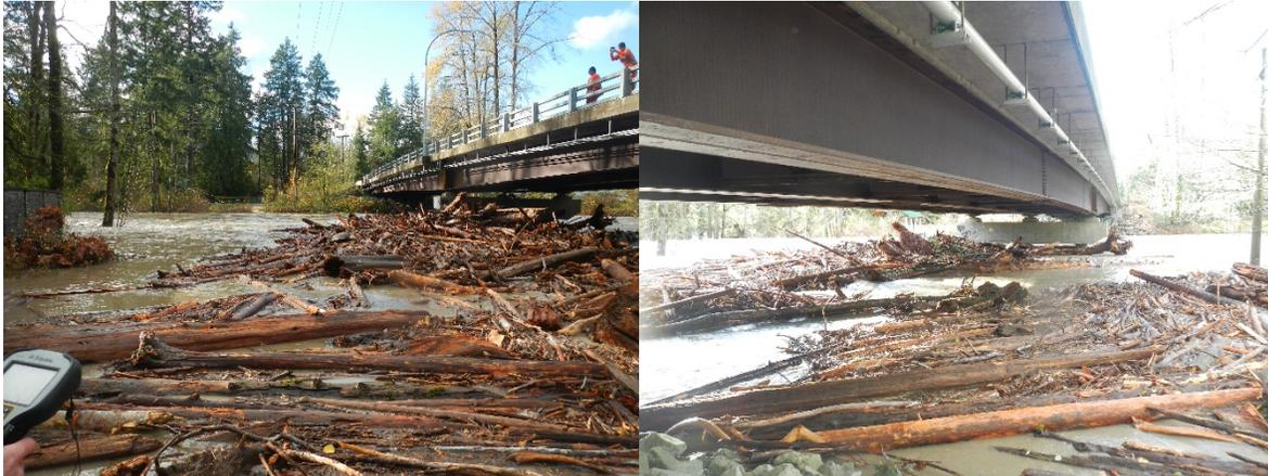
**Photo 4.2** Log jam under Hwy 1A bridge on right bank during Nov 15, 2021 flood as seen from right bank looking under bridge from upstream (left) and downstream (right) side.
