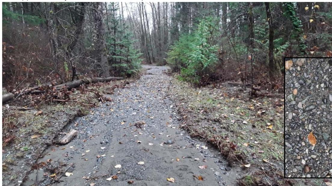
▶ Bed lowering along the left side of the channel at RK 5.8, resulting from sediment removal in 2021.
