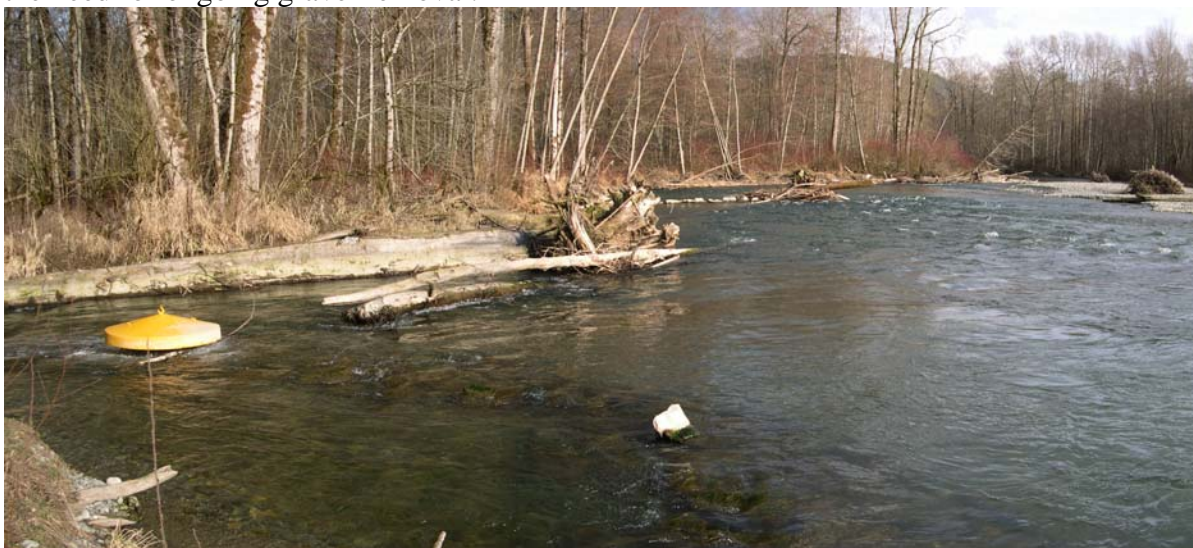
Photo 8.4: Downstream view of lower Fish Gut Alley side-channel intake showing avulsing mainstem flow and proposed installation of ballasted LWD intake feature.
