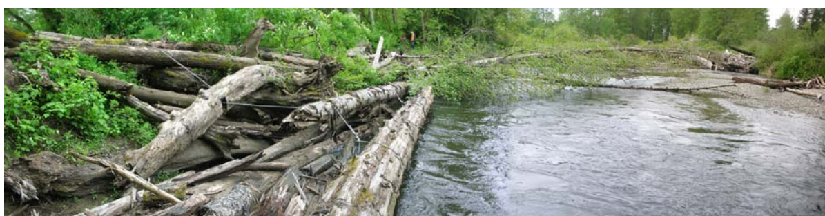
Photo 8.3 : Upstream view of log jam on Koksilah River at km 3+290
