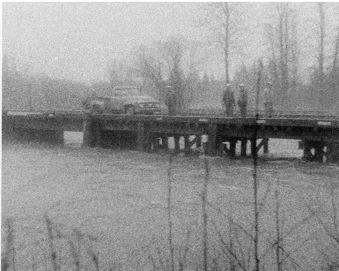
Log jam starting to form at upstream side of bridge.
