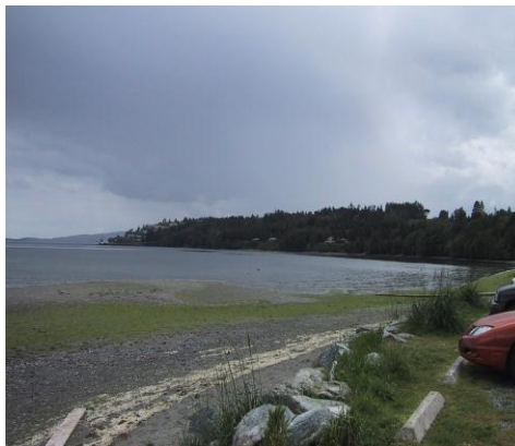
Cherry Point Nature Park in Cobble Hill currently has riprap edging along the high tide line, met by gravel parking on the other side.
