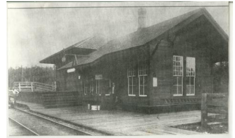
Original Cobble Hill Train Station 1906
