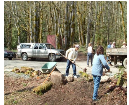
Local volunteers building the South Cowichan Off-leash Dog Park
