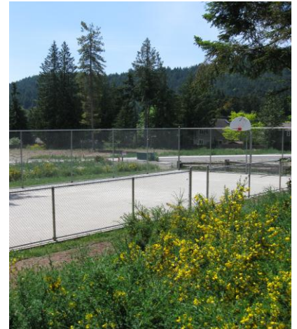
Galliers Road Park sports court surrounded by invasive Broom.
