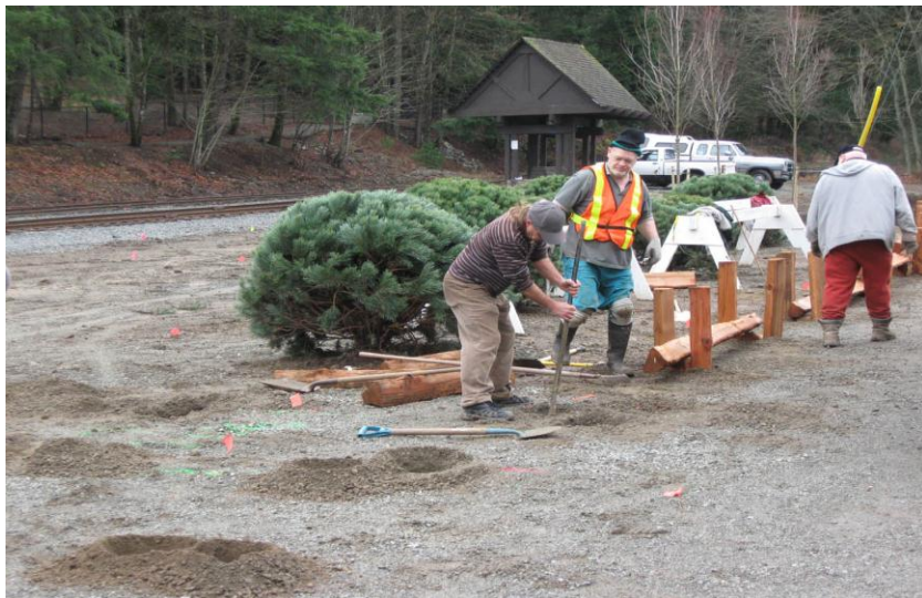
Volunteers working hard installing split rail fencing at the Train Station
