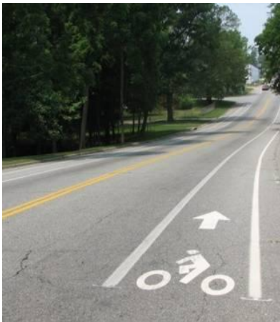
Shoulder walkways along BC MoT roadways
